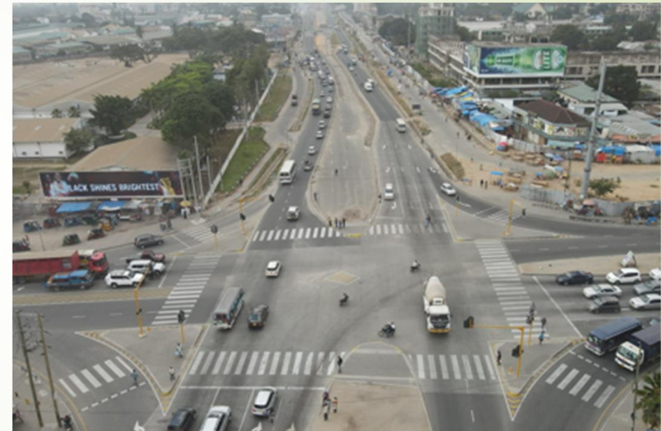
New Bagamoyo Road Widening Project
